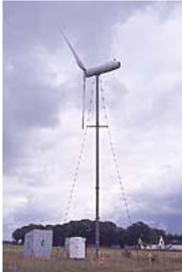
Guyed Pole Tower
