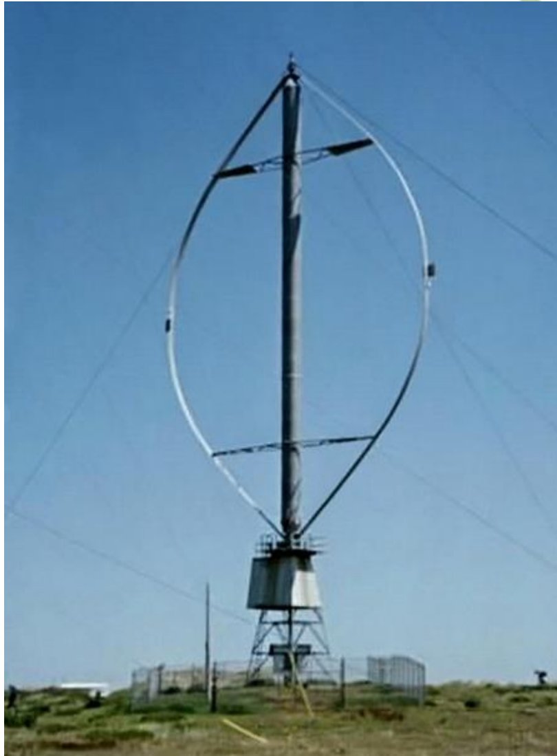
Darrieus wind turbine is vertical axis wind turbine.
