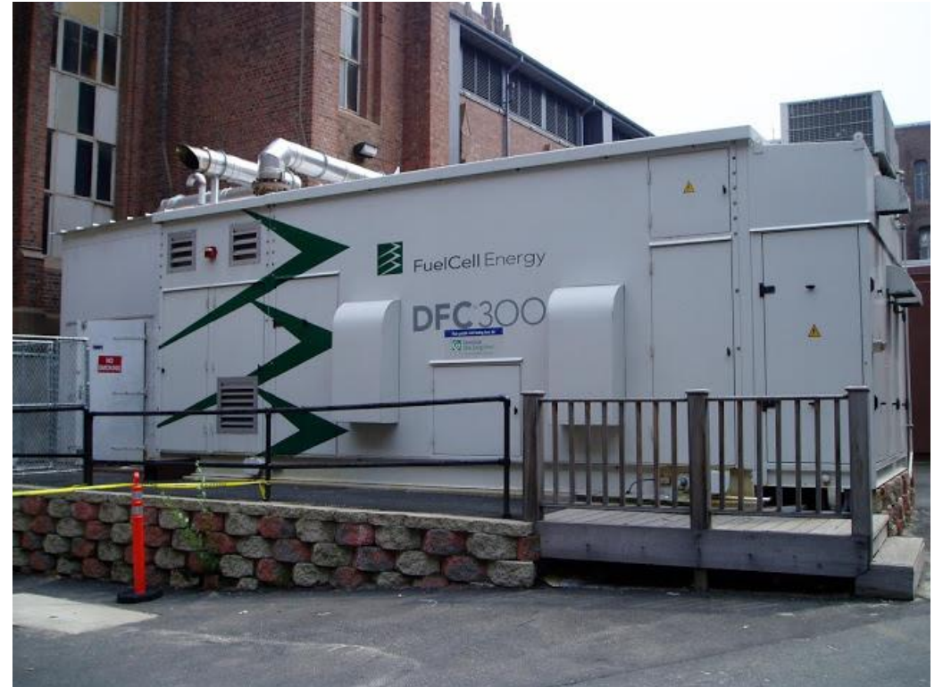
300 kW DFC 300 Fuel Cell power plant
